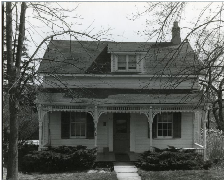
196 Widder Street East, 1980 view
